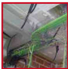
False floors and false ceilings
